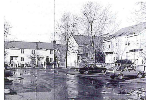
Harwell Homes, 56-units, cooperative, Section 236 financing
