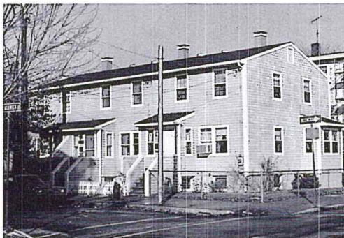
JAS Corporation, 3-units modular construction
