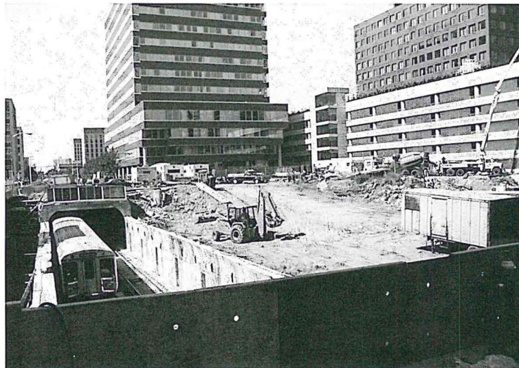
"Cut and Cover" for platform lengthening
