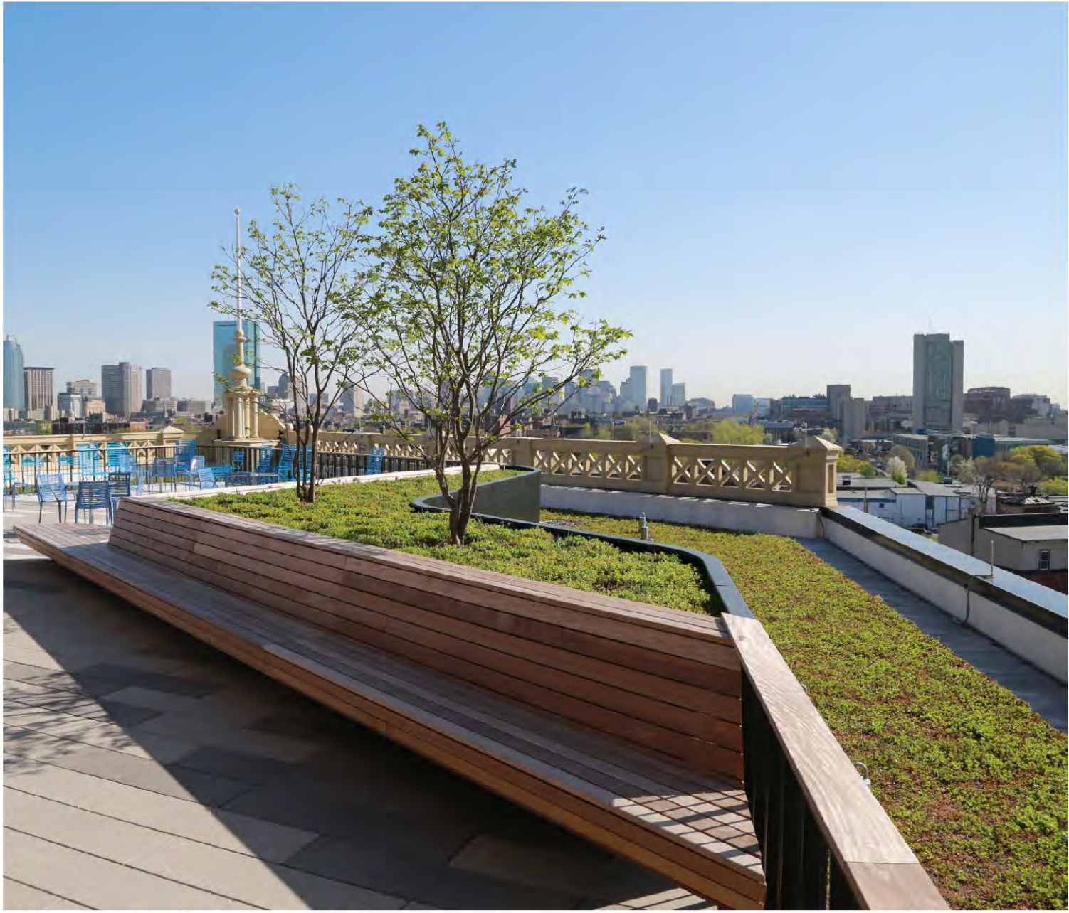
Bruce C. Bolling Municipal Building– Boston, MA
