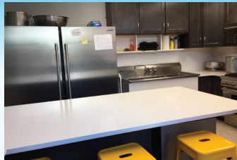
East End House Kitchen Renovation (2016)
