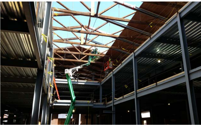
Installation of new roof wood decking
