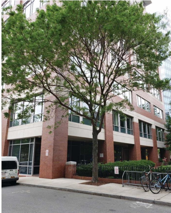
East Facade - Existing
