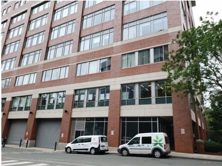
South Facade - Existing
