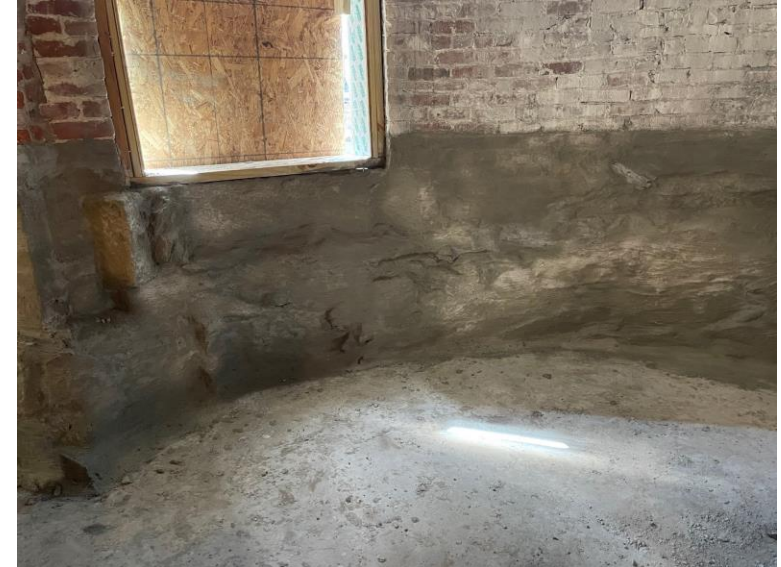
Waterproofing / masonry restoration
