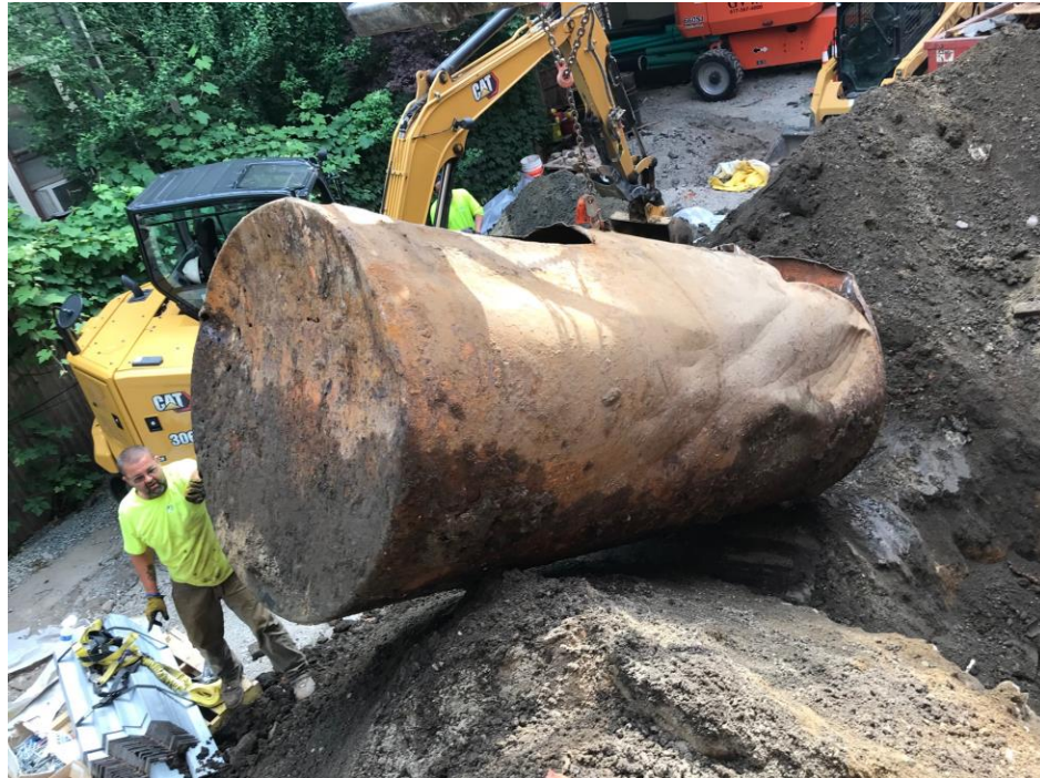
Oil Tank Removal
