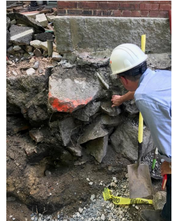
Stone Foundation Reconstruction
