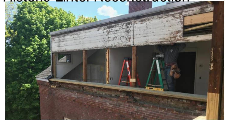
Historic Lintel Reconstruction
