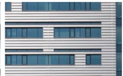
Introducing solid wall cladding embeds the scale of occupants and interior spaces on the elevations in addition to allowing for complementary materials to the urban context.
