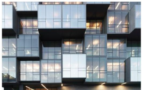
Above: Reveals and recesses in the facade breakdown the proportions of large facades. Below: Plane changes on the facade allow opportunities for exterior spaces and introduce a smaller scale of inhabitation on the facade.
