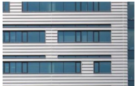
Introducing solid wall cladding embeds the scale of occupants and interior spaces on the elevations in addition to allowing for complementary materials to the urban context.
