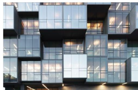
Above: Reveals and recesses in the facade breakdown the proportions of large facades. Below: Plane changes on the facade allow opportunities for exterior spaces and introduce a smaller scale of inhabitation on the facade.
