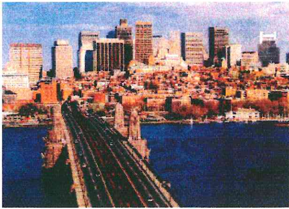
The Longfellow Bridge
