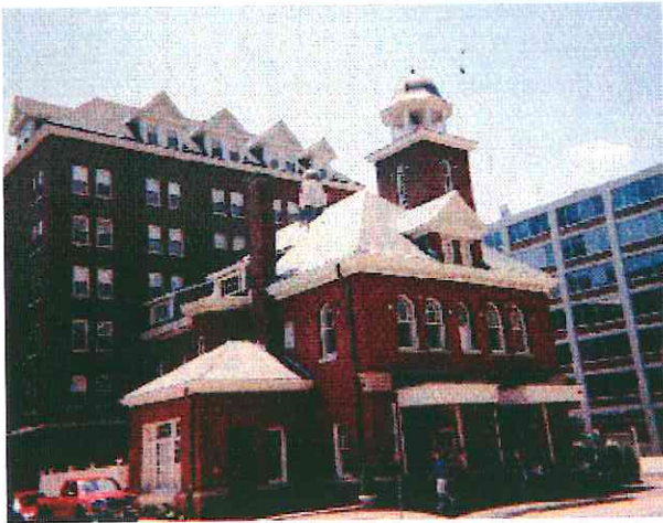
The Kendall Hotel post construction.
