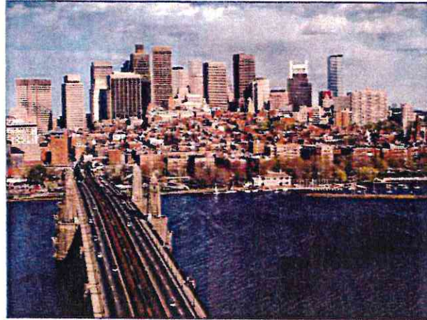
Longfellow Bridge, Cambridge, MA
