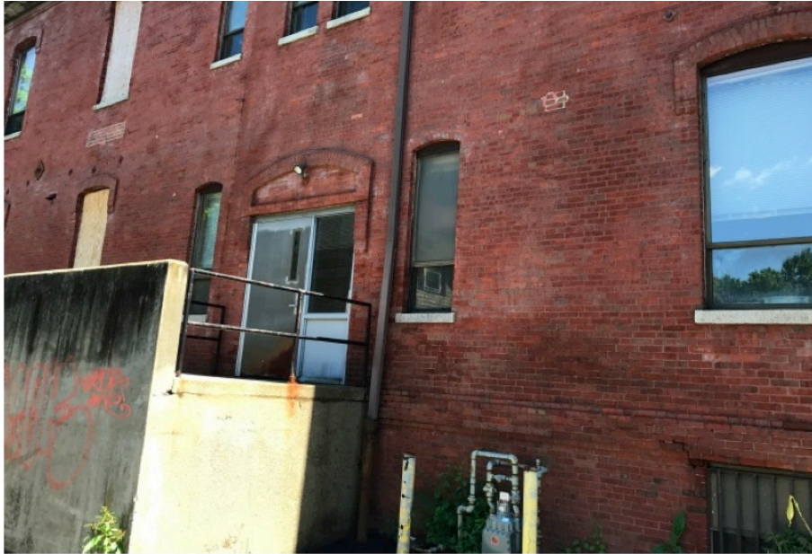
EXISTING REAR ENTRANCE
