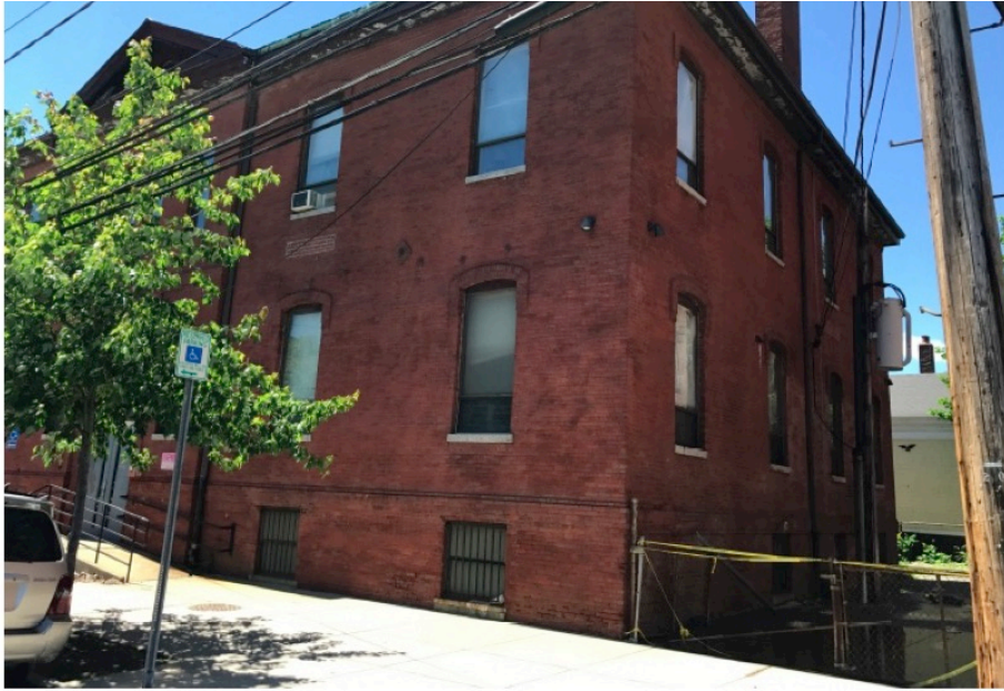
EXISTING FRONT FACING RIGHT CORNER
