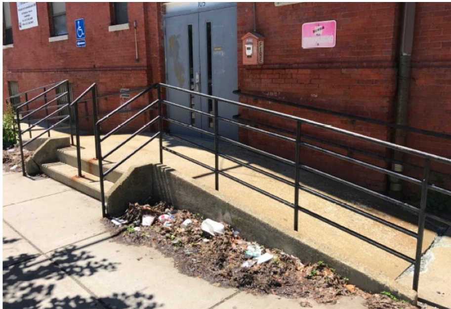
EXISTING FRONT ENTRANCE
