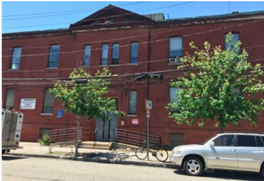
EXISTING FRONT OF BUILDING
