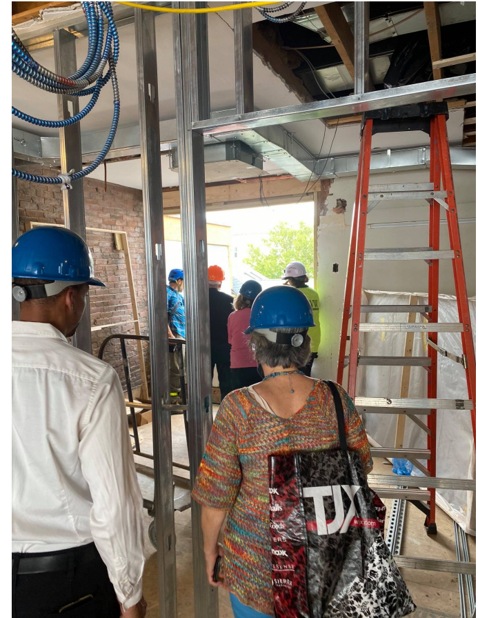
95-99 Bishop Allen Construction Site
