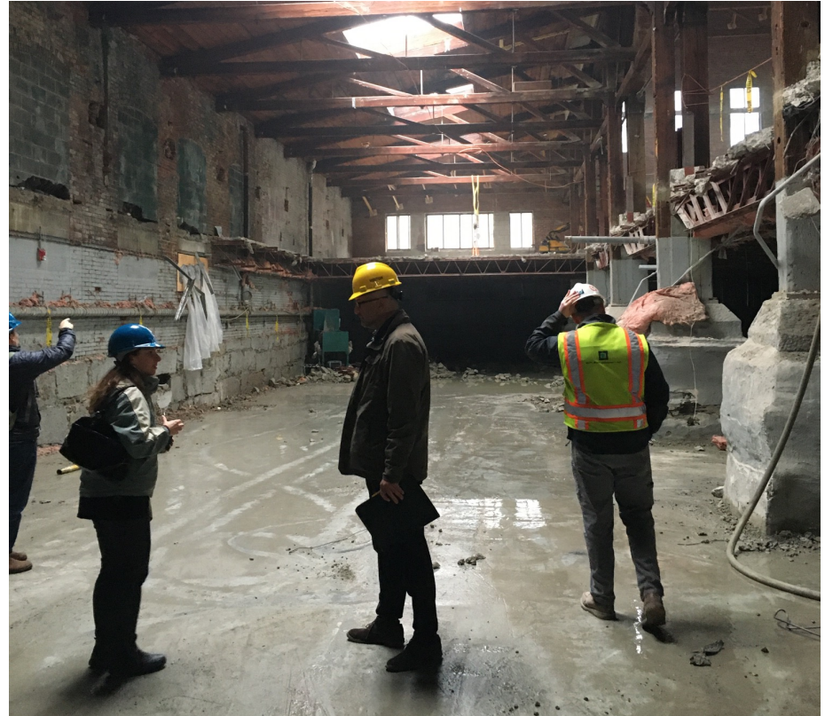
Foundry Construction Site
