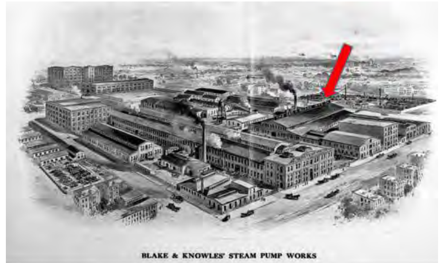
Petition for Historic Landmark Status
