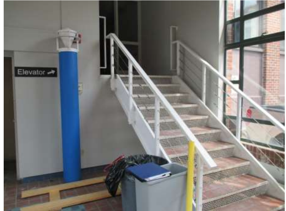
Existing first floor is approximately 5 feet above street level, which inhibits gathering and assembly uses
