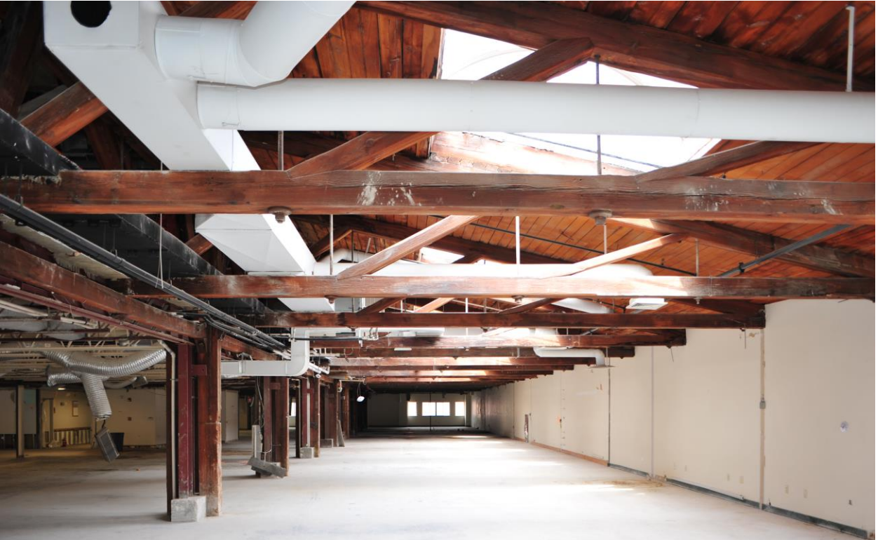
101 Rogers Street, first floor. Roof framing under side aisle.
