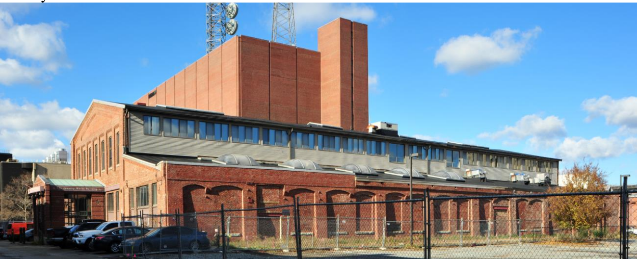
101 Rogers Street, east elevation
