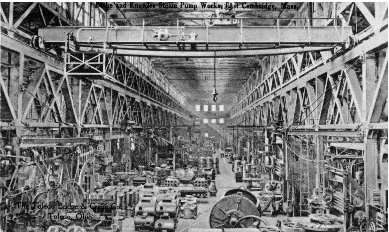
Interior of the Blake & Knowles machine shop showing the timber framing and craneway. This building was designed and built by the same firm as the Foundry, two years later. CHC postcard collection.
