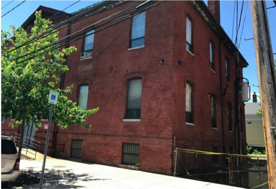
EXISTING FRONT FACING RIGHT CORNER
