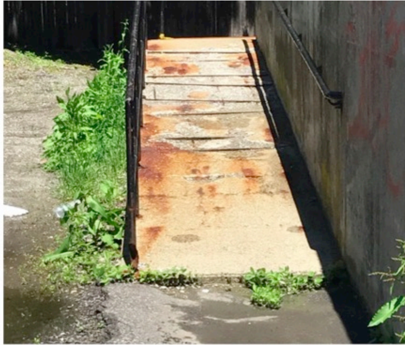
EXISTING REAR HANDICAP RAMP
