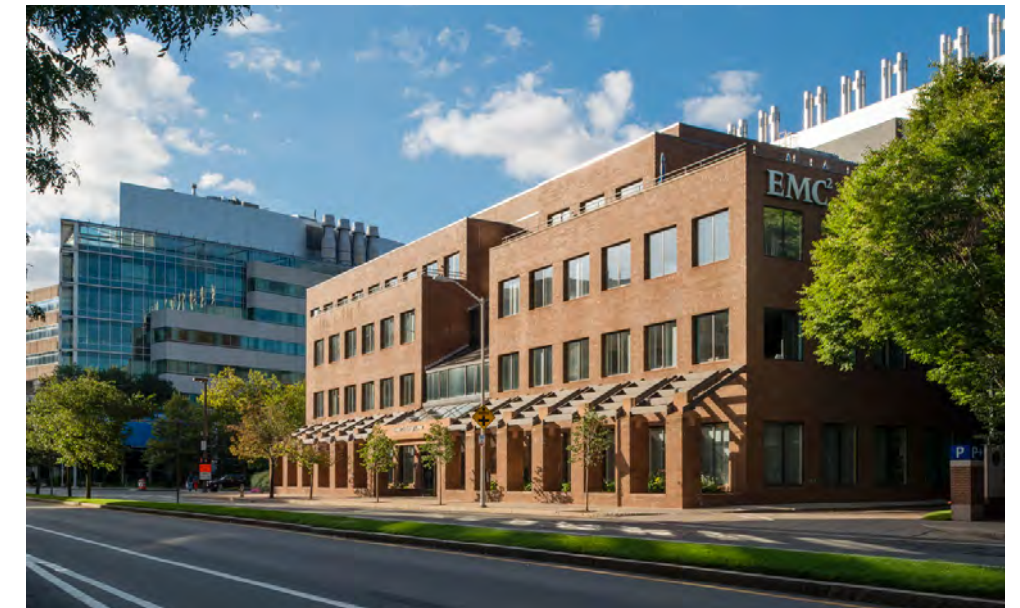
1. Existing Site Photo
