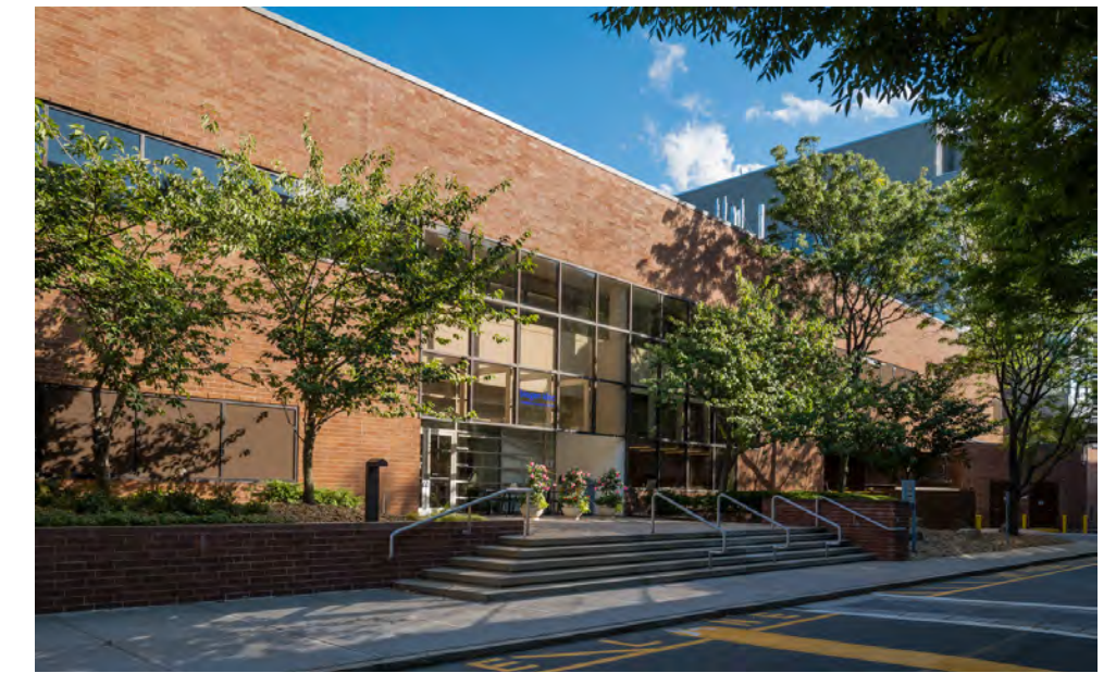
1. Existing Site Photo
