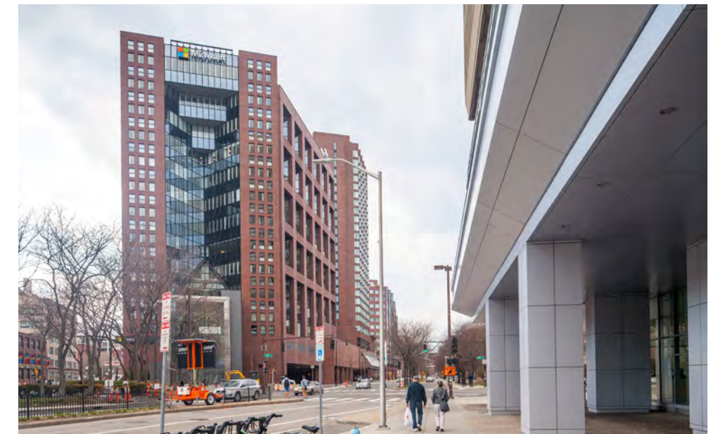
1. Existing Site Photo
