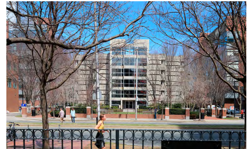
1. Existing Site Photo
