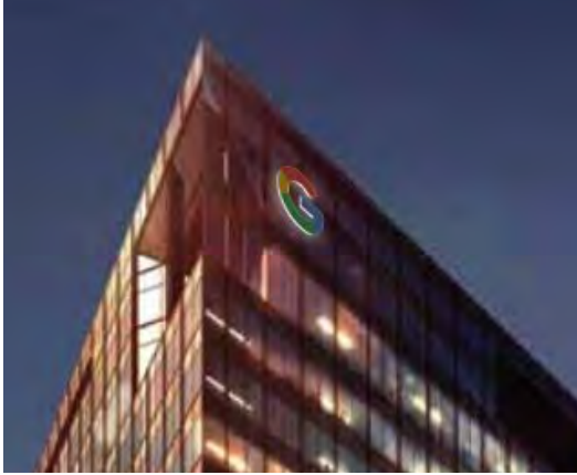
15' diameter G; recessed edge lit sign, note front face of sign is not illuminated
