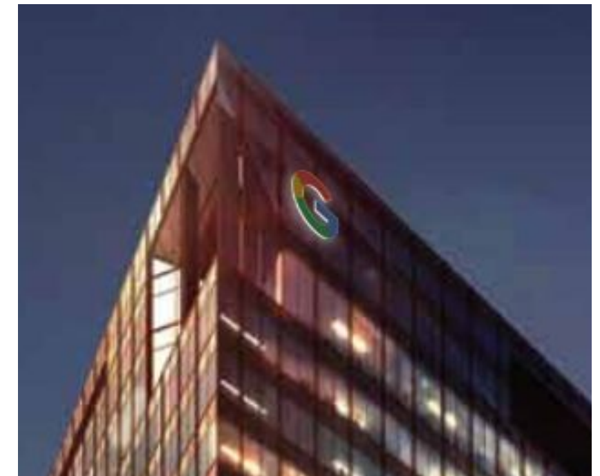
15' diameter G; recessed edge lit sign, note front face of sign is not illuminated
