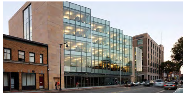
The Novartis Institutes for Biomedical Research | Permitting, Site/Civil Engineering, Survey, LEED Certification Support
