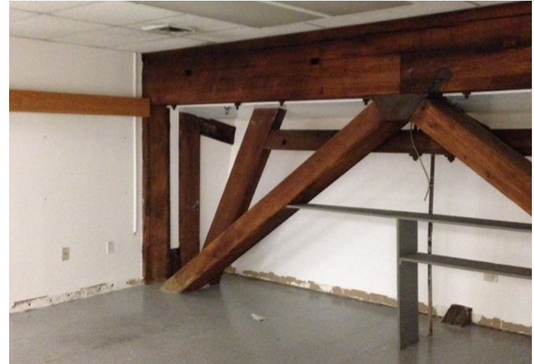
Existing Foundry space
