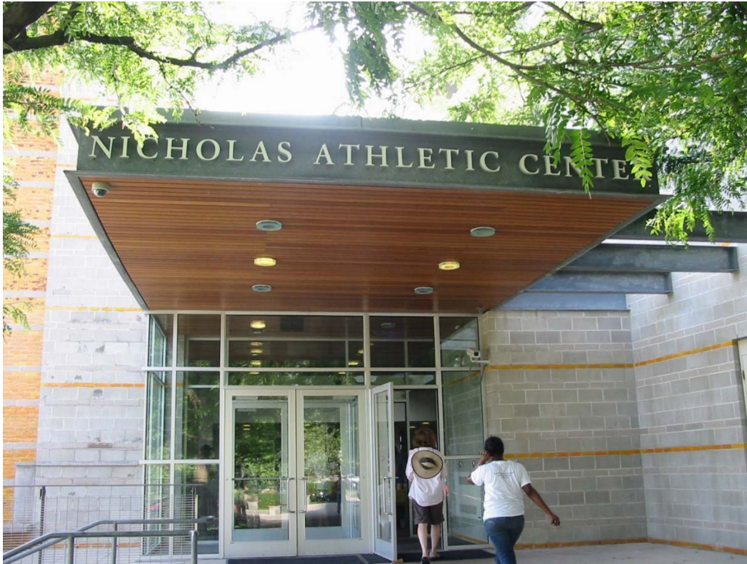
Subtle variation in the CMU base. (Buckingham Browne and Nichols Field House, Cambridge, MA.)
