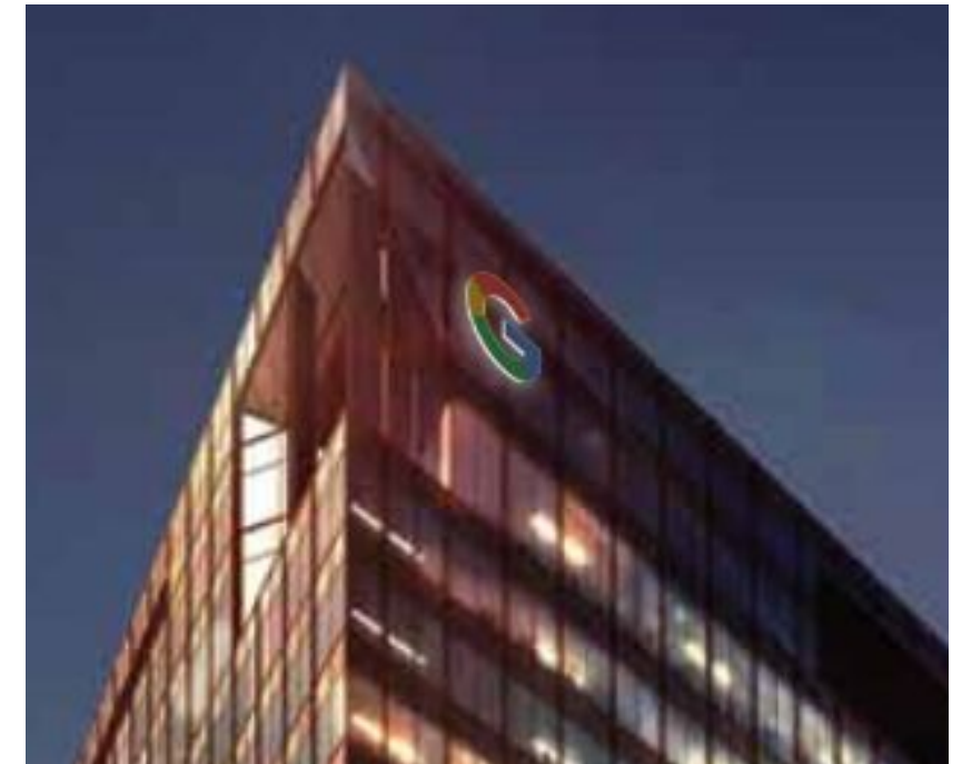
15' diameter G; recessed edge lit sign, note front face of sign is not illuminated
