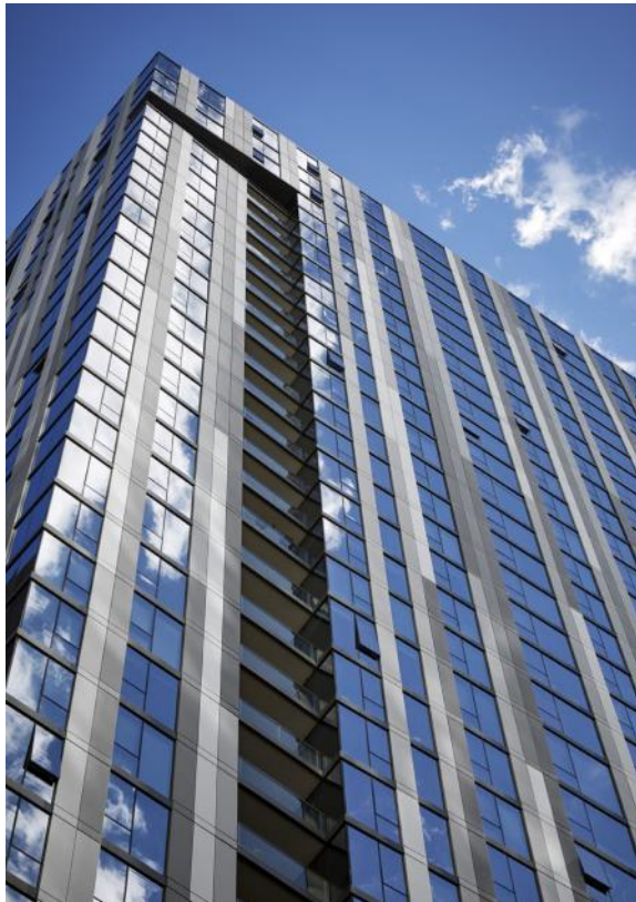
Inset balconies create visual interest and relief in large facades helping to break down the scale of the building as well as providing an outdoor space for residents to enjoy.
