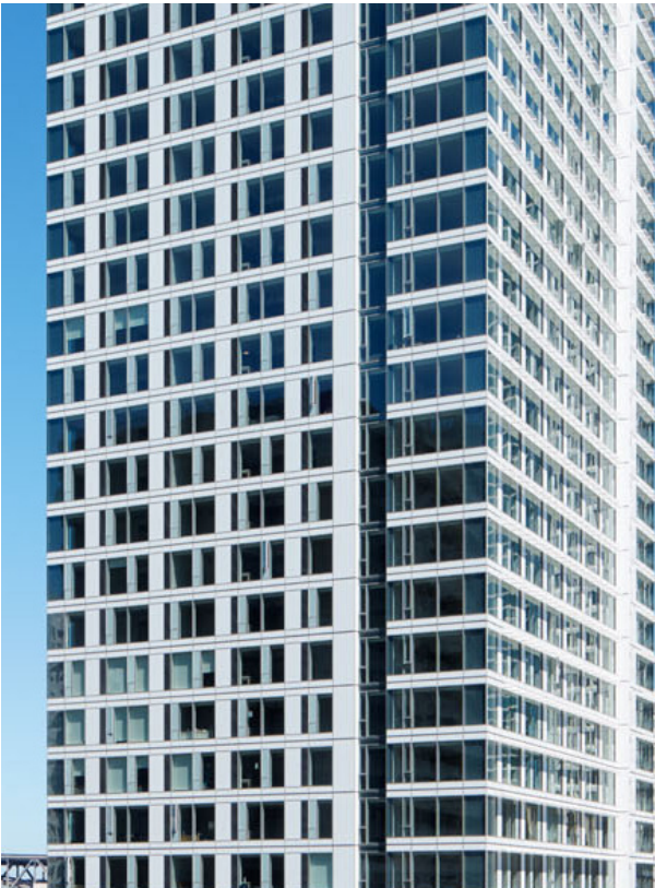
Horizontal spandrels and other pattern facades can be used to accentuate thinner proportions within the building. These strategies work in combination to break down the scale of the mass.
