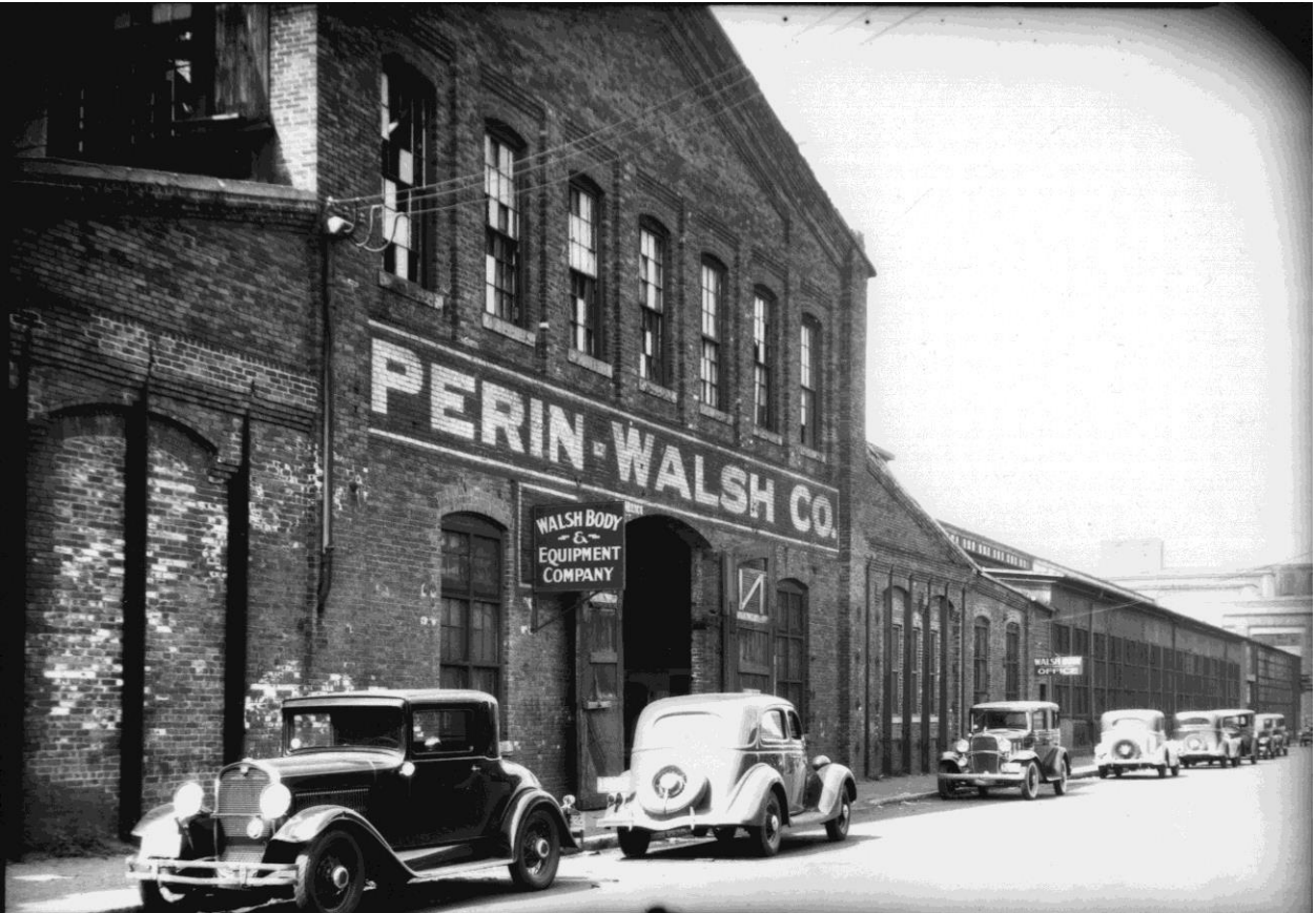
101 Rogers Street, Bent Street elevation, 1935
