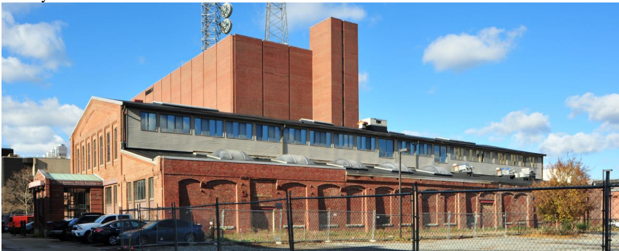
101 Rogers Street, east elevation
