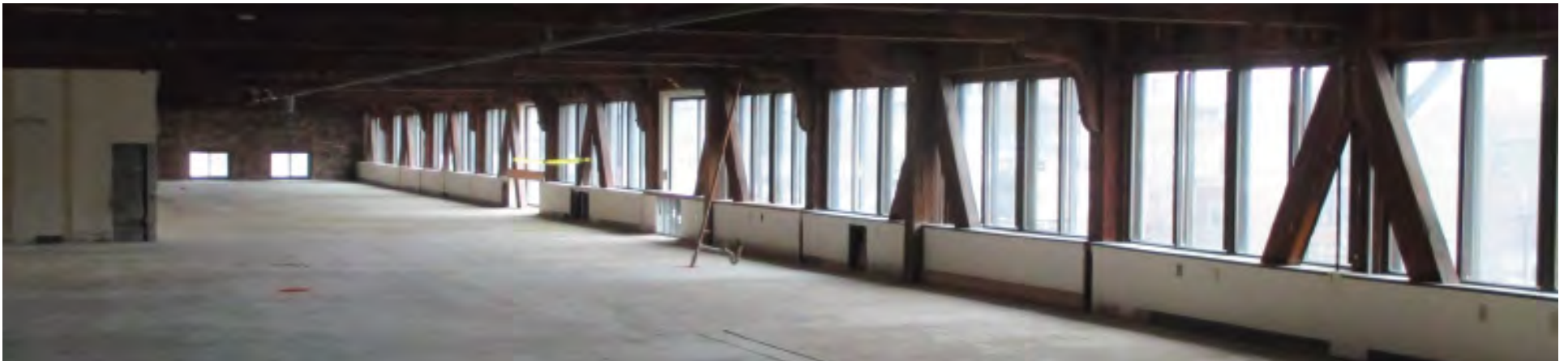
Existing interior space on the 2nd floor
