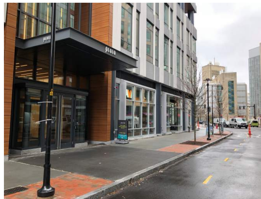
Columns west of 88 Ames entrance, with wraps removed.
