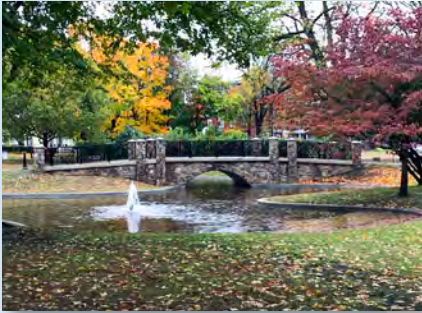
Farlow Park Bridge and Pond Restoration, Newton, MA
