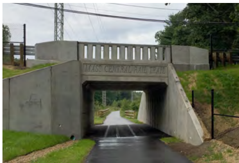
Mass Central Rail Trail, Weston Rail Trail Underpass, Weston, MA
