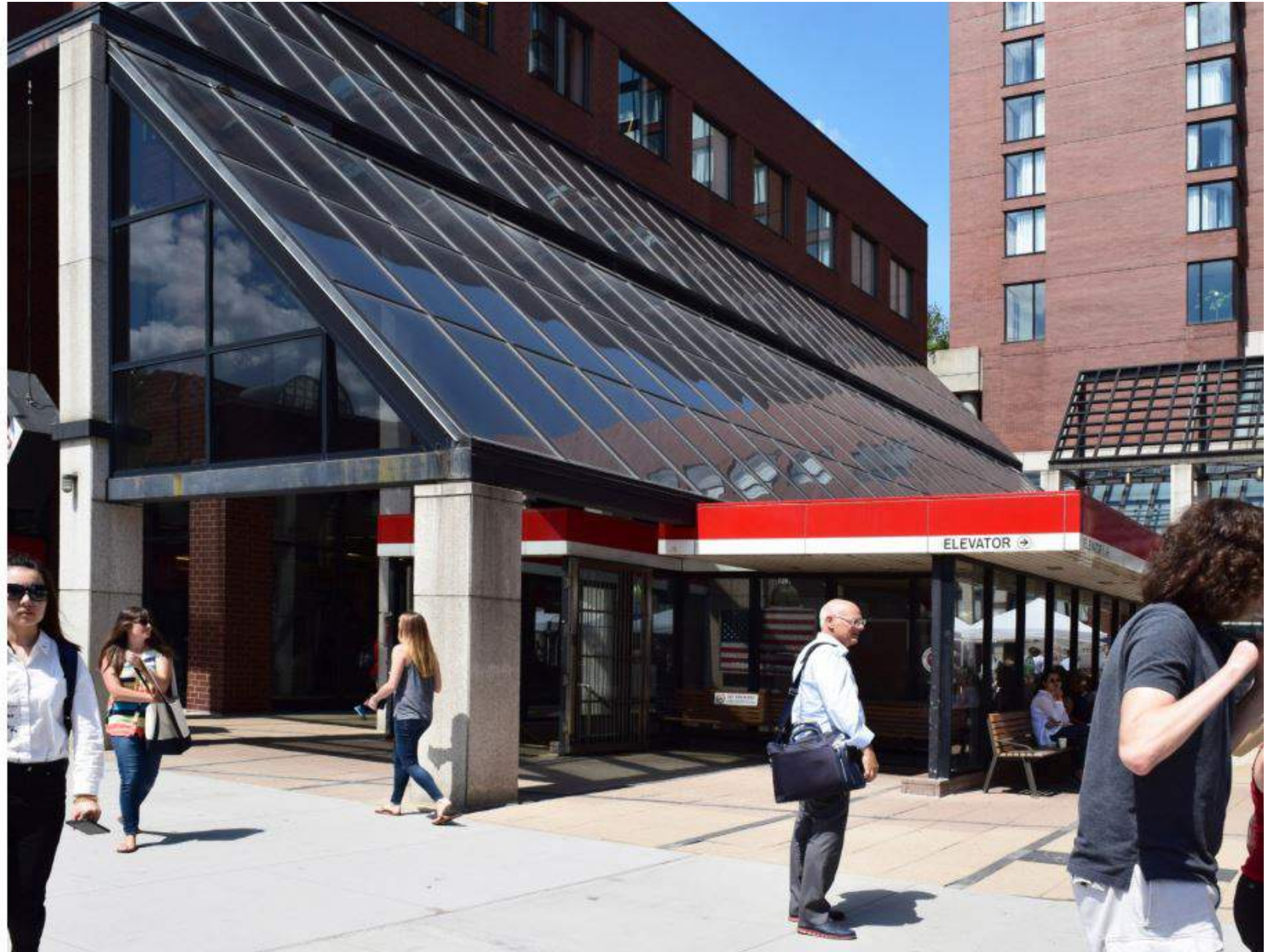
EXTERIOR VIEW LOOKING AT MAIN STREET ENTRANCE
