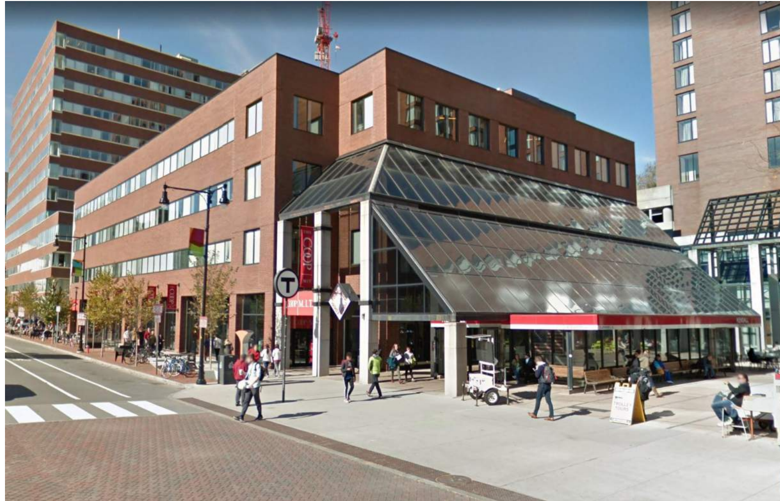
SOUTHEAST CORNER OF 325 MAIN STREET BUILDING
