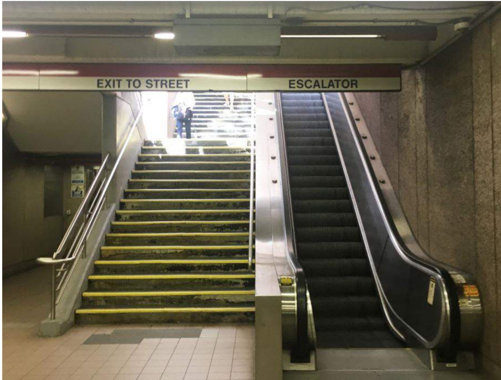
INTERIOR VIEW FROM TRACK LEVEL
