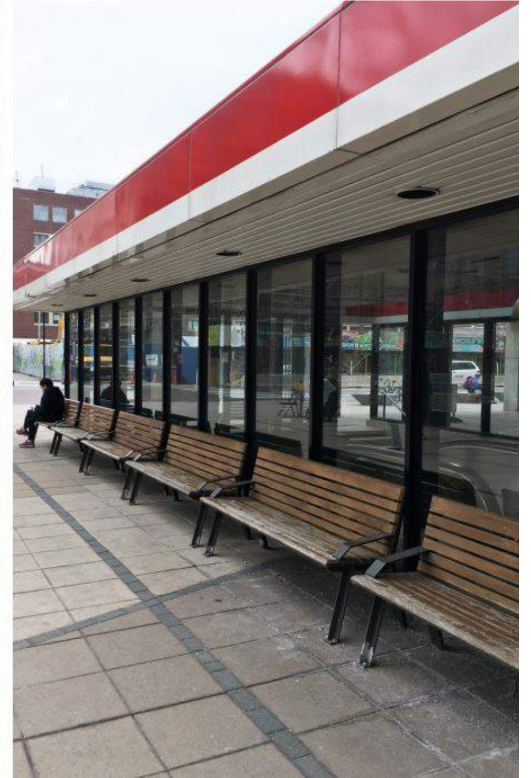
EXTERIOR VIEW DEPICTING EAST FACADE AND BENCHES
