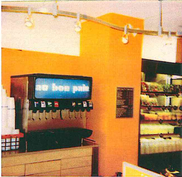
Renovations at Au Bon Pain in the Food Court
