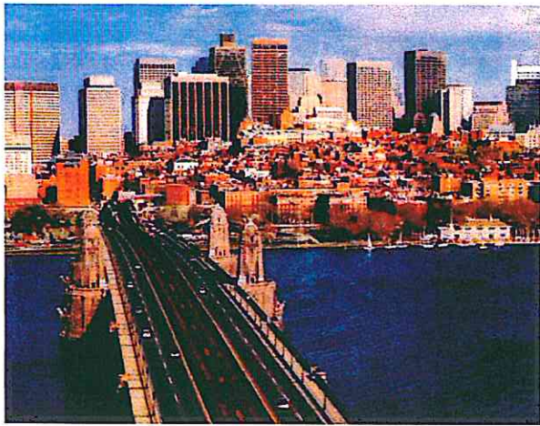
The Longfellow Bridge
