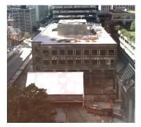
325 Main Street's abatement of the brick façade, which was found to contain non-friable asbestos, is now complete. Structural demolition of the building is anticipated to start in mid-October, and be complete by mid-November. The wing-wall for 325 Main Street's Visual Mock-Up is on track to be installed by the end of this month. 325 Main Street's Phase II Design Documents were received electronically on Monday, September 16<sup>th</sup>. The set is being checked for completeness.
