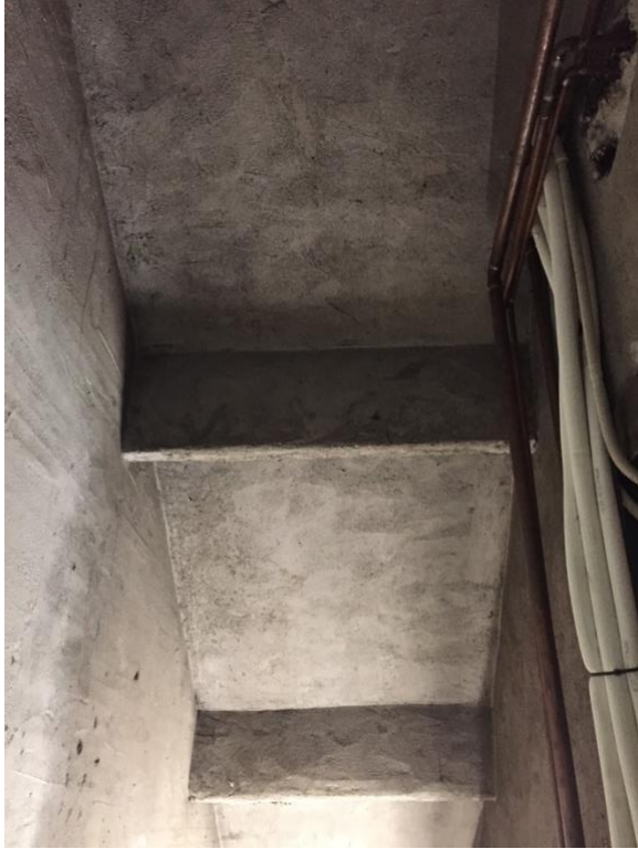
Underside of the staircase where structural support work is beginning, July 2020
