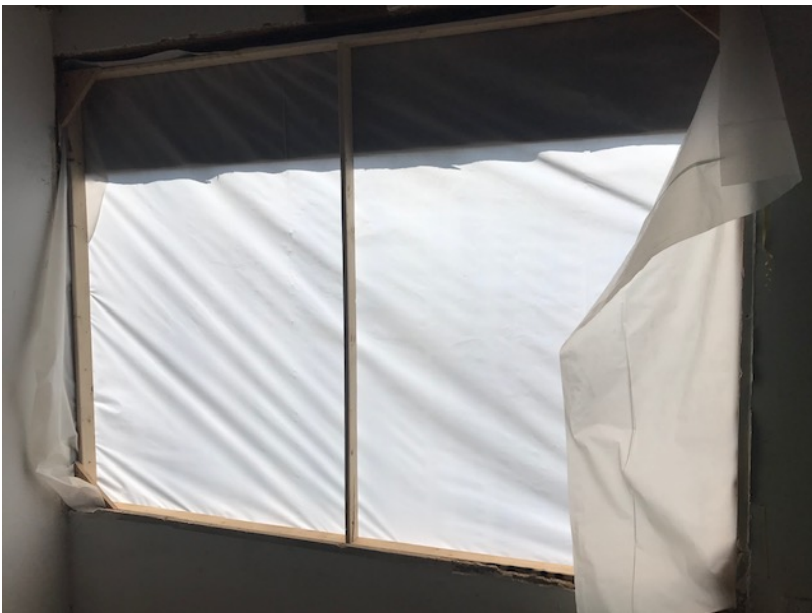
Left: Protective covering installed after removal of dormer window Right: wall partitions
