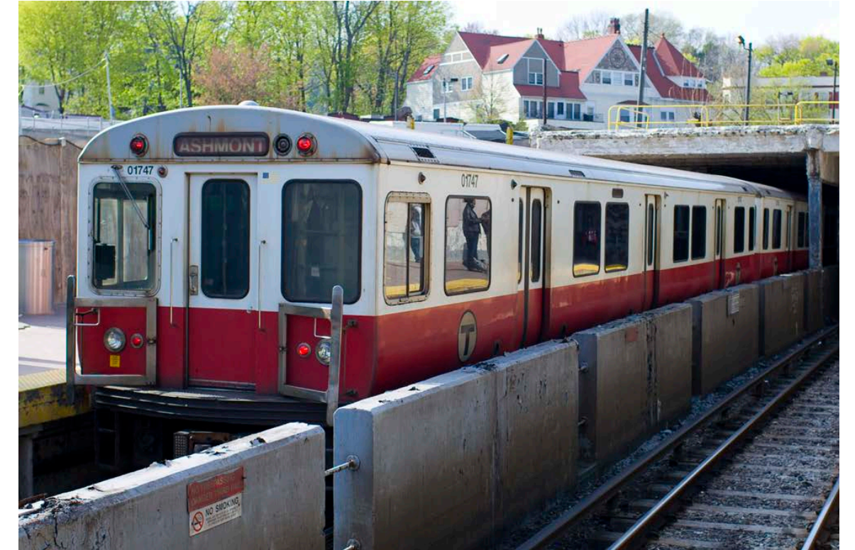
Types of Equipment: Underground Rail Tunnel
