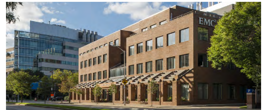
Existing Site Photo
