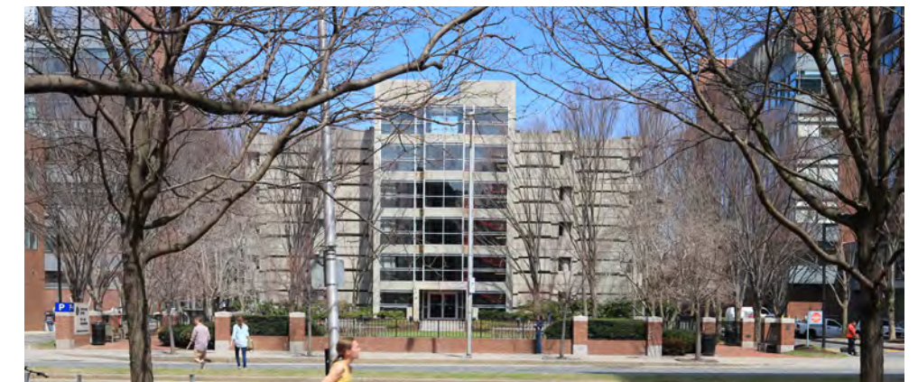
Existing Site Photo
