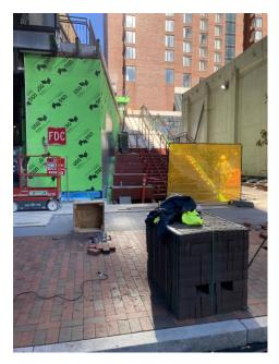
As part of the 325 Main Street project, Main Street itself is taking shape. The pedestrian barricade has been removed to allow for repaving. The concrete sidewalk has been poured, trees have been planted, and crews are installing brick pavers. Entry canopy and soffit work along the facade edge of the building are still underway. BXP intends to reopen a portion of the Main Street sidewalk in the next few weeks.
